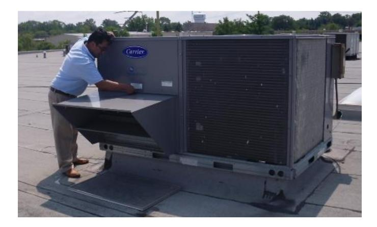
Two RTUs are single-stage heating/cooling units while four RTUs are two-stage heating/cooling units with economizers. All six units are scheduled using a variety of headends for testing purposes.
